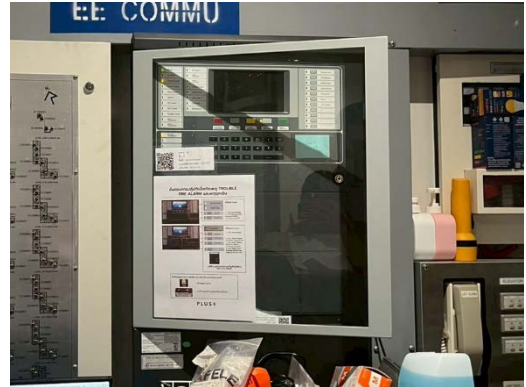
Fire Alarm Control Panel
