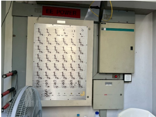
Fire Alarm System Graphic Annunciator
